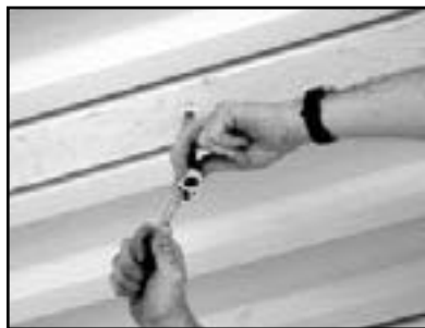
Figure 11: Installing the hanger bolt
